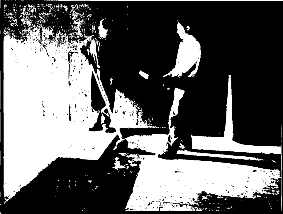
THE LAYING-ON OF ROCK CORK
